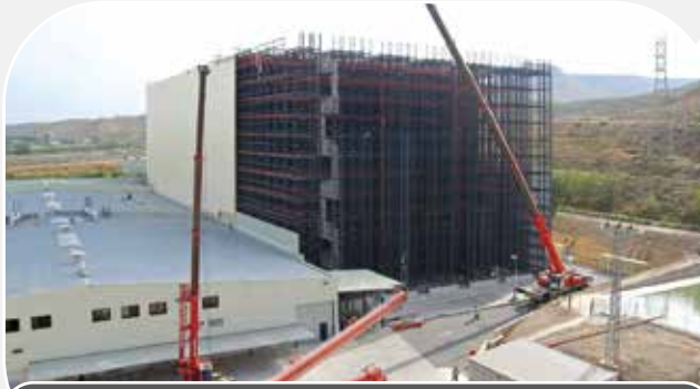
Self support (Rack-support building)
