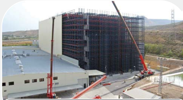
Self support (Rack-support building)
